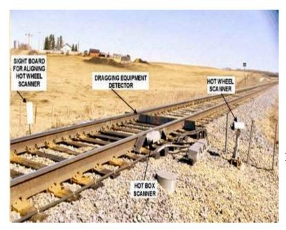
Crews cannot reliably hear the report of wayside defect detectors when trains grow to excessive lengths. When that happens, the train must often stop and follow procedures to make sure their train is safe to proceed.
